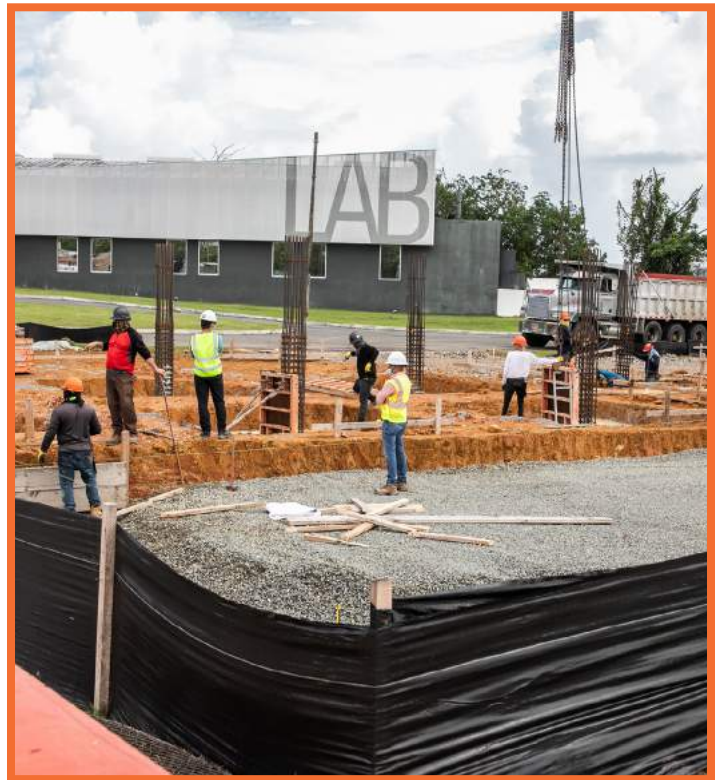
Forward Center Construction Process
