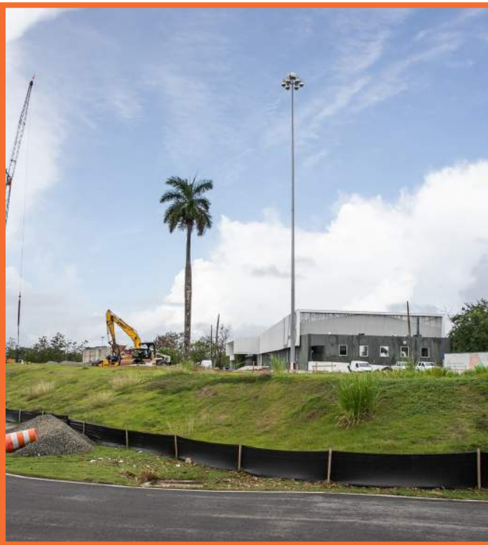
Forward Center Construction Process
